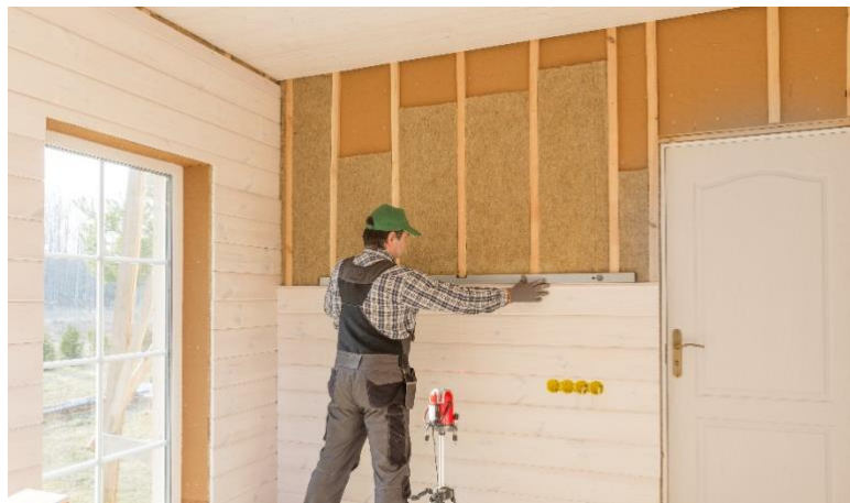
Fig 3. Hemp fibres used in building insulation
